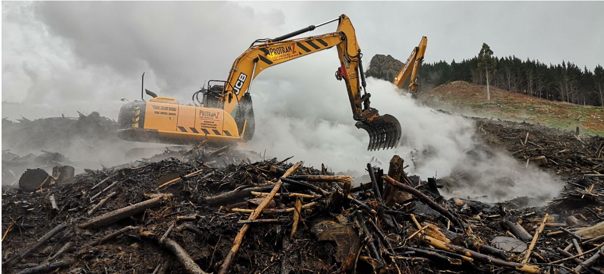
Image 2. Example of an excavator with root rake (B. Janes, FENZ. Packhorse Hut, Gebbies Pass).
